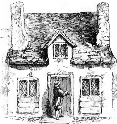
BUNYAN'S HOUSE AT BEDFORD.
